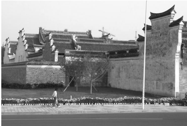
Figure 9. Collapsed Walls after Remedy
