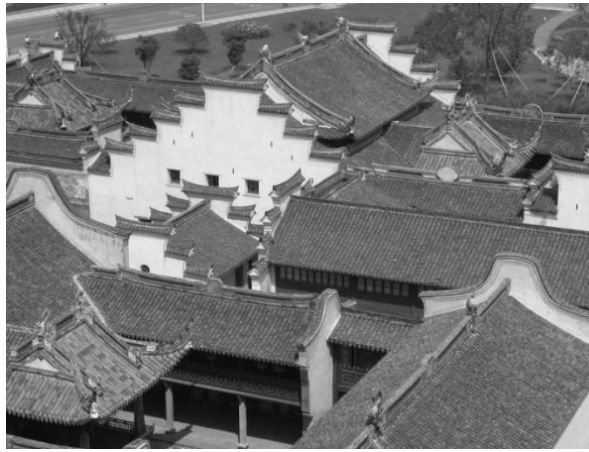
Figure1. Status quo of the Hall Source: Taken by Team Members of Research Program
