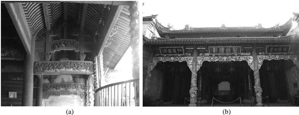
Figure 4. Roof Upward View: (a) Internal Roof; (b) External Roof
