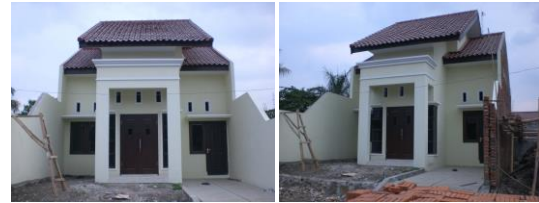
Gambar 8. Nirwana Sulfat Residence.
