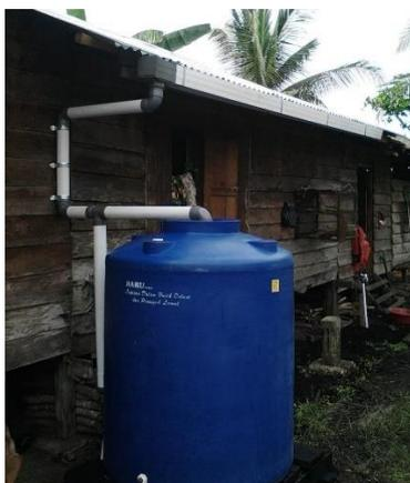
Figure 6: The main component rainwater harvesting system
