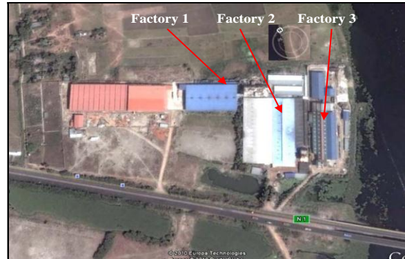
Figure 1. Location of three adjacent factory buildings
