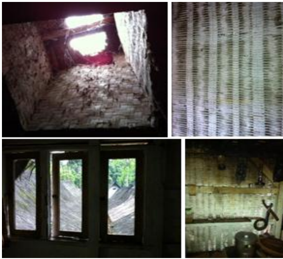
Fig. 3. The use of day lighting in chimney, woven wall, and openings in Kampong Naga Local House
